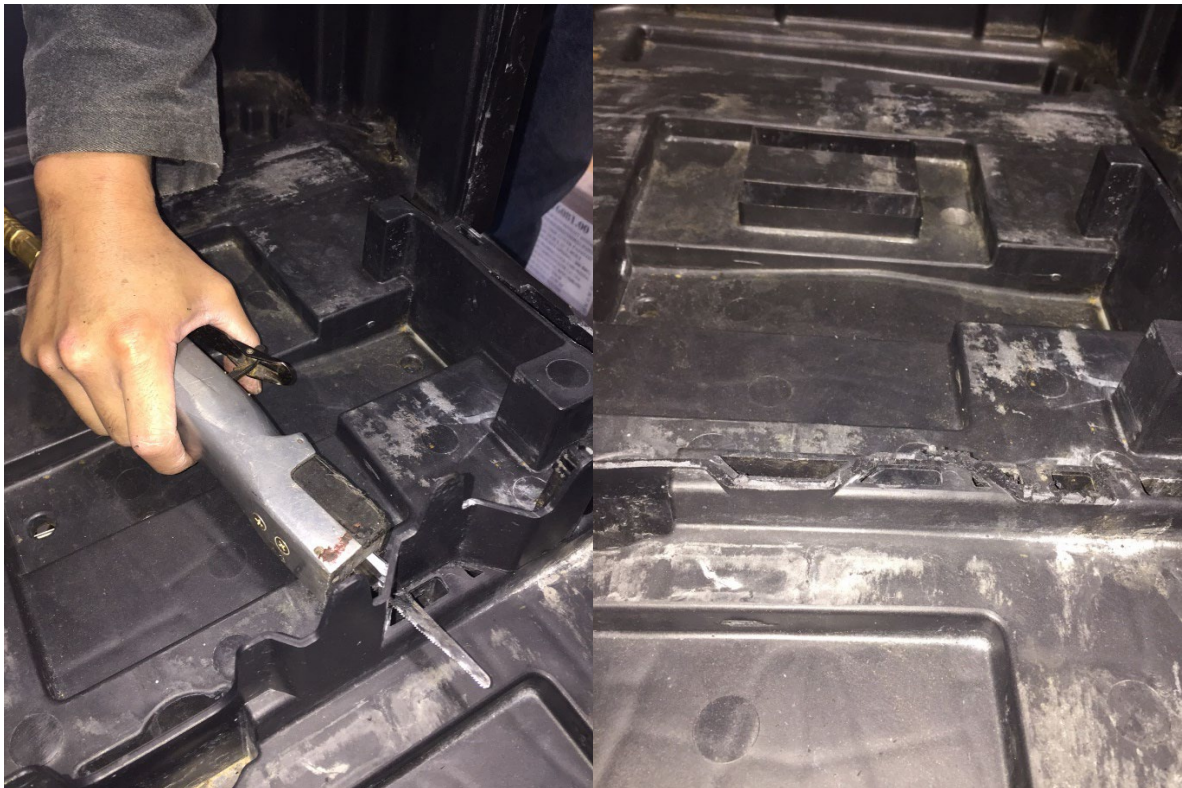
Fig. 6- Raised material removed.
